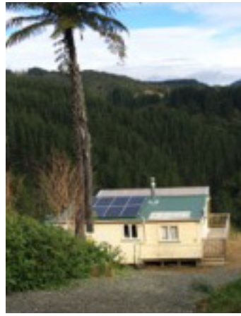
Solar panels power much of the hut.
